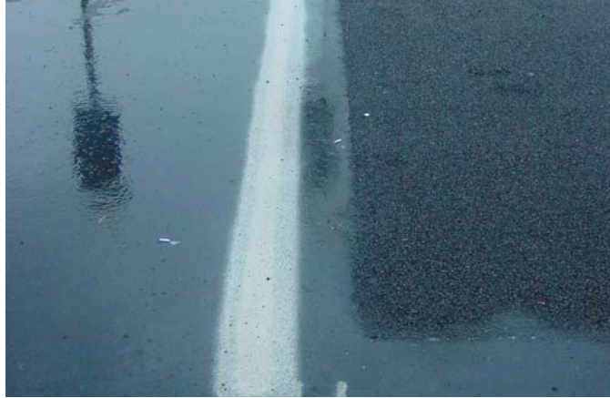
Figure 18. A comparison of traditional asphalt (left) and porous asphalt (right) when wet. The gaps created by leaving out the finer particles in porous asphalt allow water to infiltrate pavement and into the structural soil reservoir below. As a result, porous asphalt appears dull when wet, because water runs through and does not pond, which creates a high friction surface.
