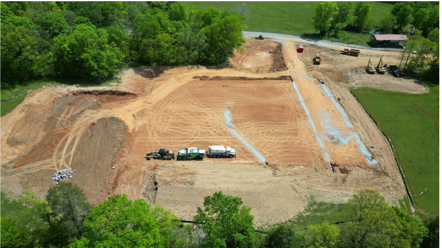
PSTC – Burn Tower Site & Utilities
